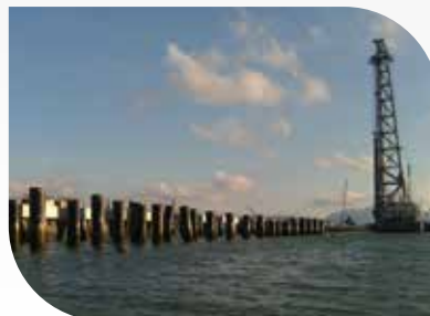
Shenhua Coal Terminal Port, Zuhai, China
