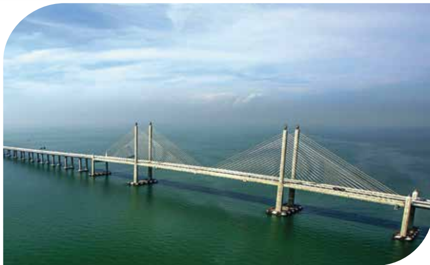
2nd Penang Bridge, Penang, Malaysia
