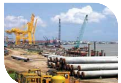
One Kilometer Container Terminal, Chittagong Port, Bangladesh
