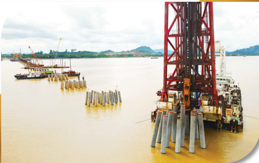
Batang Lupar Bridge, Sarawak (90m length pile prejoined in ICP factory)
