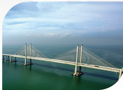
2nd Penang Bridge, Penang, Malaysia
