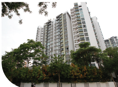
Park Green Condominium, SengKang East Ave, Singapore
